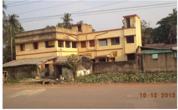
Hospital CH-NO.39+200 LHS
